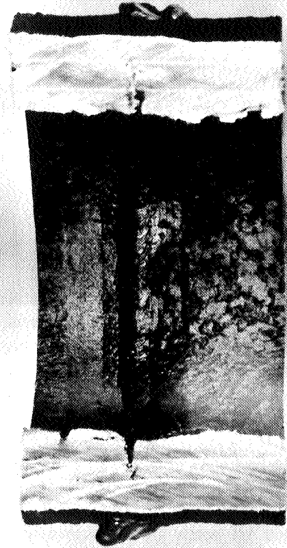
Figure 2. Circumferential Rupture Through Weld
